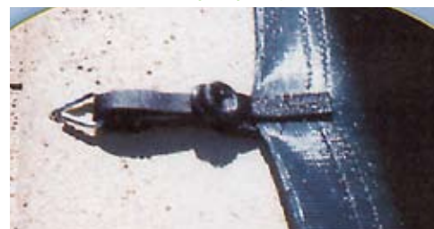
Flush mounted anchors
